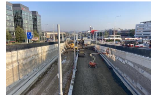
New tram line – the biggest investment in public transport in Brno in the last 20 years
